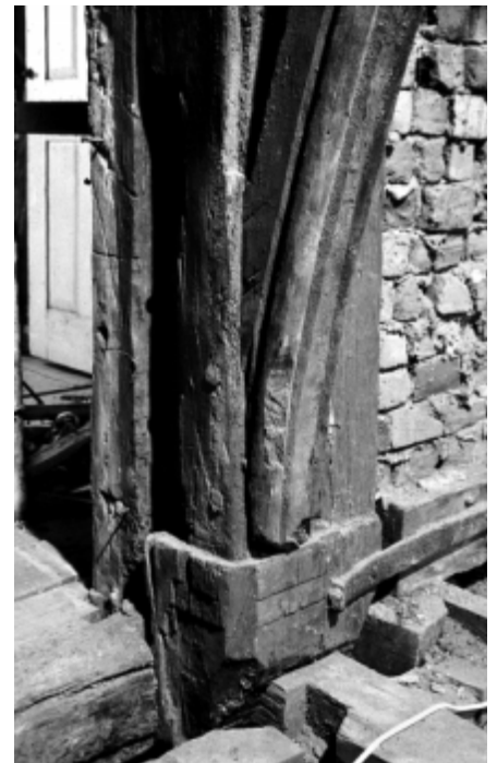
▲ Detail of east arcade-post.
