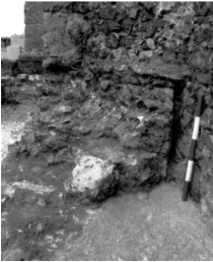
▲ Detail showing later church masonry sitting over earlier foundations, looking east. Scale 0.5 m.
