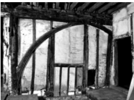
▲ East arcade of hall infilled with later sixteenth-century framing and window.
