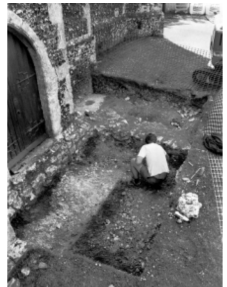
▲ Earlier wall foundations exposed in front of the north door.
