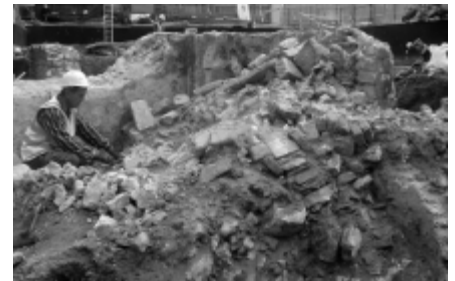
▲ Excavating the friary demolition rubble from within the warming room.
