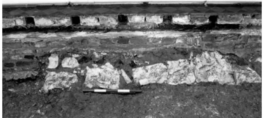
▲ Detail of the north nave wall foundation exposed during the replacement of the later spring floor. Scale 0.5 m.
