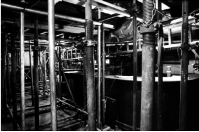
▲ The public bar made safe with temporary props.
