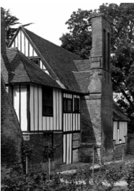
▲ Rear elevation of drawing room range showing base of earlier sixteenth-century chimney.
