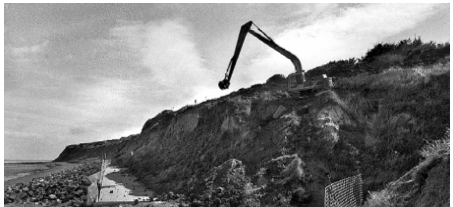
▲ Machine work in progress.
