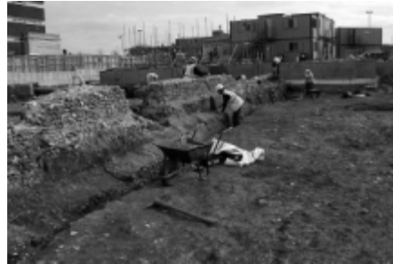
▲ Excavation along the line of the friary boundary wall.
