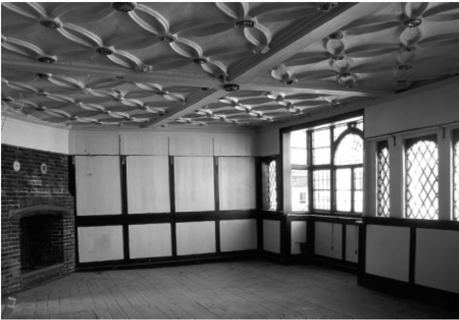
▲ First-floor chamber with decorated plaster ceiling.
