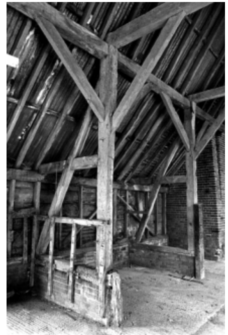
▲ Interior of timber-framed barn.
