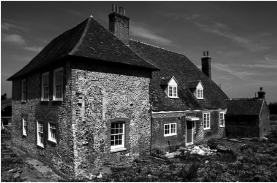
▲ View showing cross-wing in foreground and former aisled hall at the rear.
