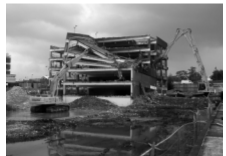
▲ Demolition of the multi-storey car park, August – September 2002.
