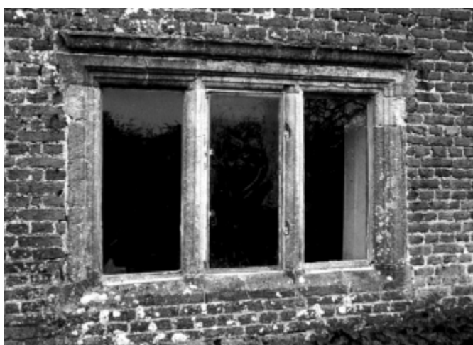
▲ Detail of ovolo-moulded stone-mullioned window.
