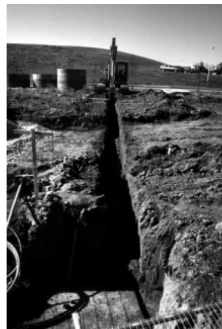
▲ Machine-cutting one of the deep service trenches.
