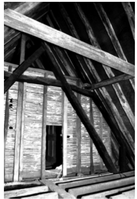
▲ Remains of original soot-blackened roof truss.
