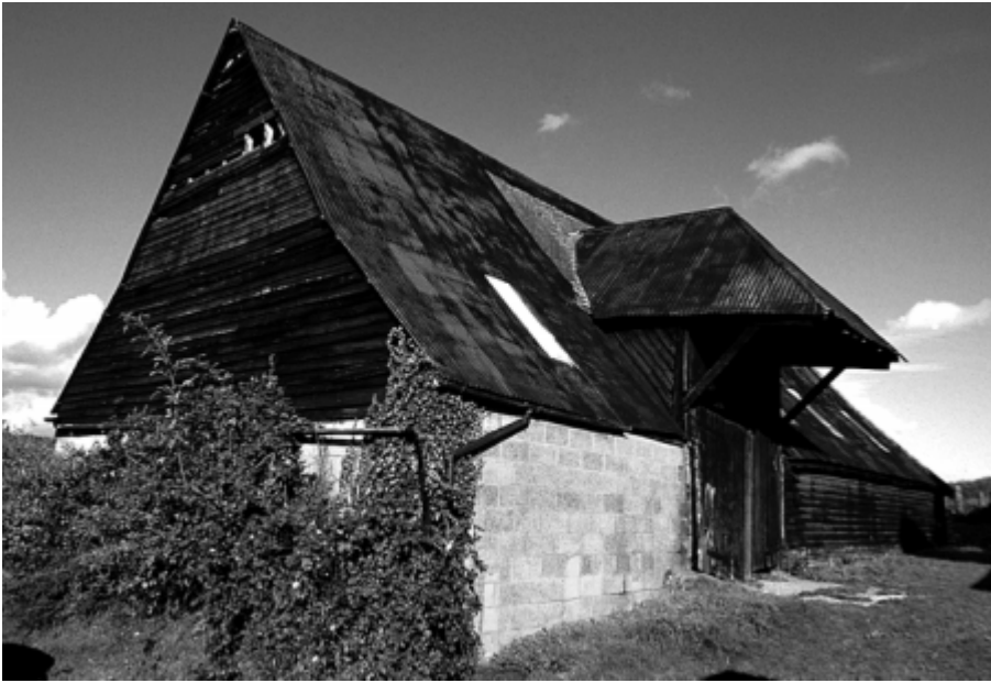
▲ General view of exterior of the timber-framed barn.
