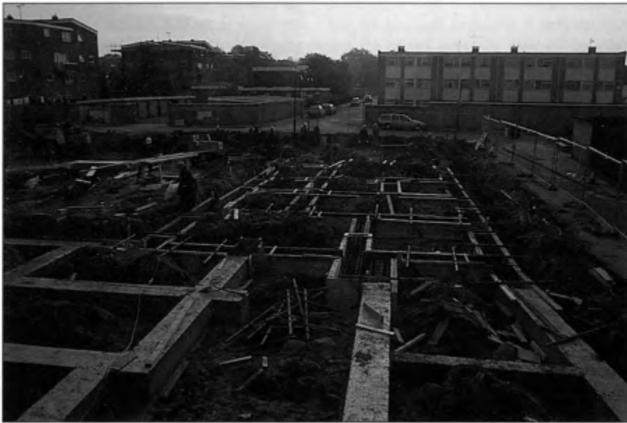
Construction work in progress.
