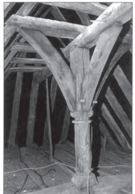
Crown post in roof space over cross-wing.
