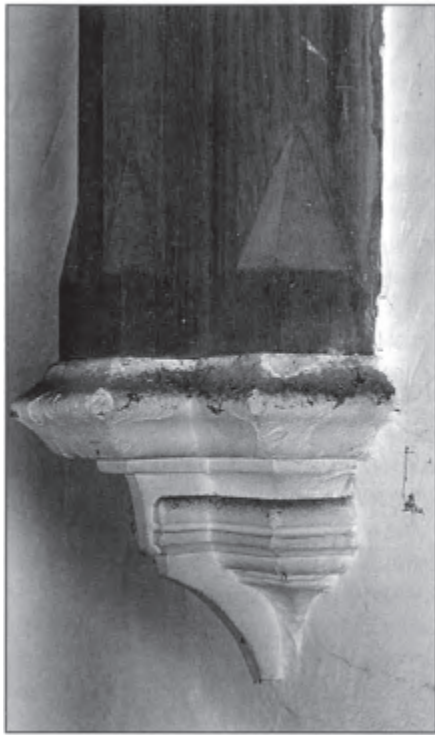
Above: Corbel detail. Right: Fifteenth-century gatehouse roof.
