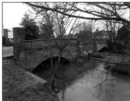
St Radigund's Bridge looking west.
