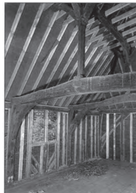
Interior of timber-framed upper chamber.
