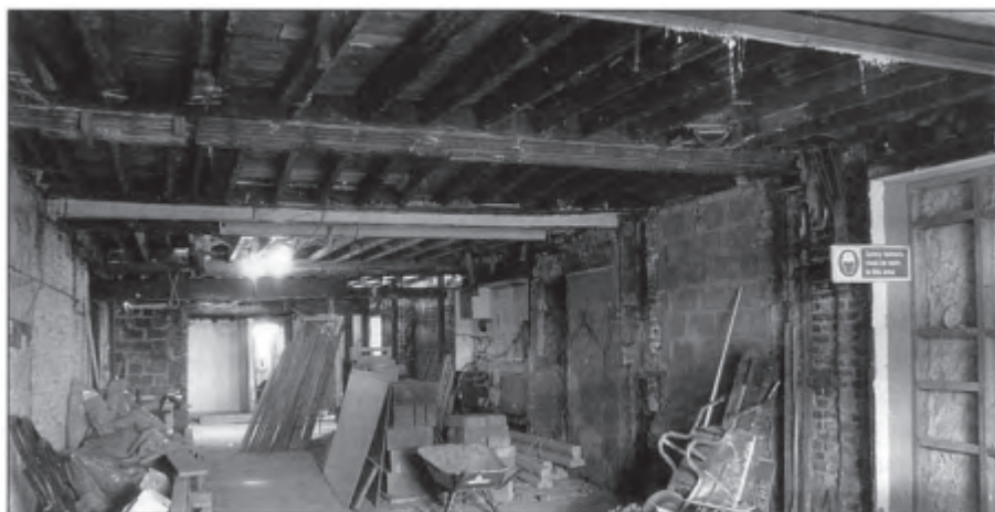
Ground floor during works showing exposed medieval joists.
