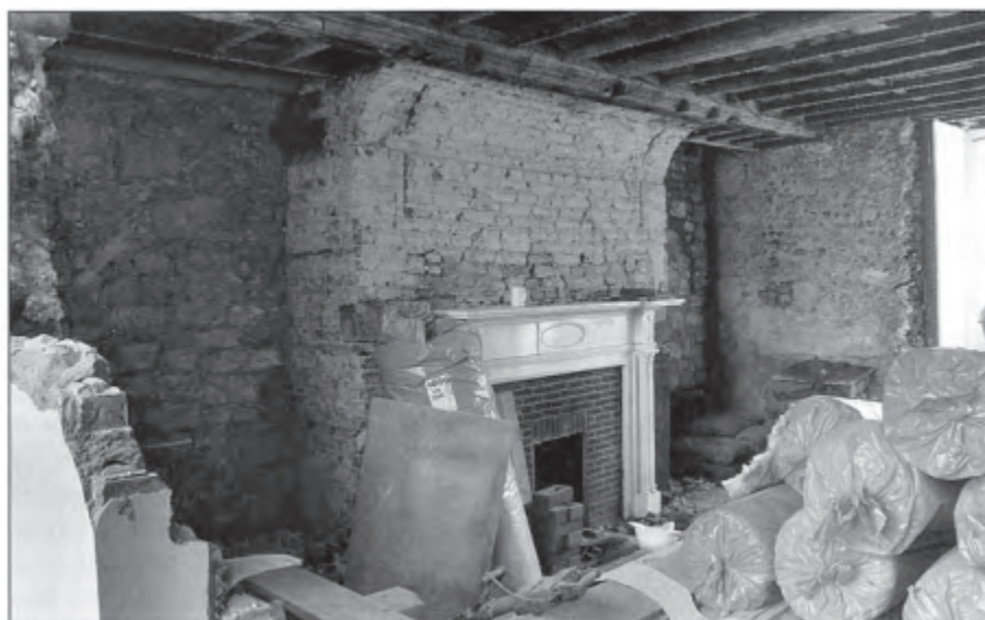
Ground floor, east end, after stripping out.
