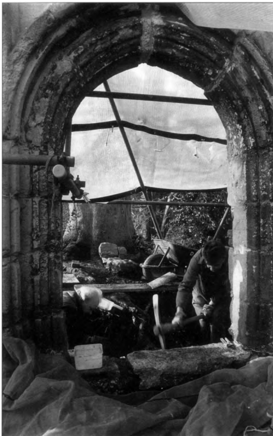
Greyfriars Gate: Works in progress (John Boulden and Alan Pope).
