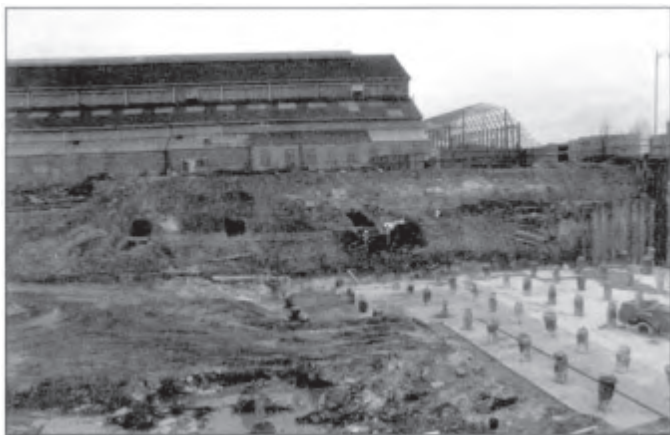
The site, looking north.
