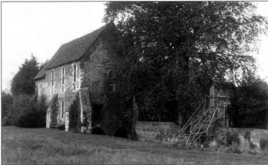
General view showing the gate and the refectory at Greyfriars.
