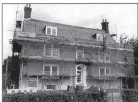
Frontage during refurbishment.
