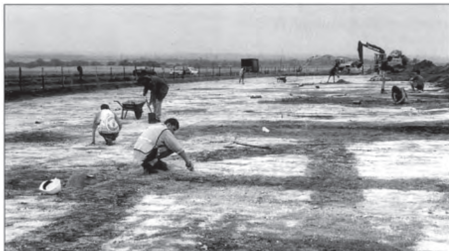
The topsoil strip in progress with exposed features being defined prior to mapping. Area 4 looking east.
