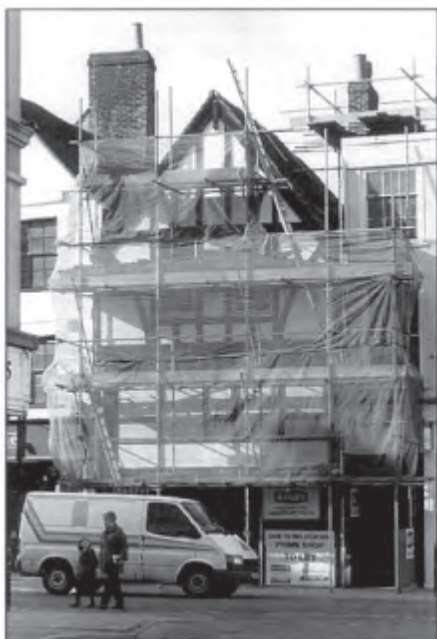
Frontage during refurbishment.
