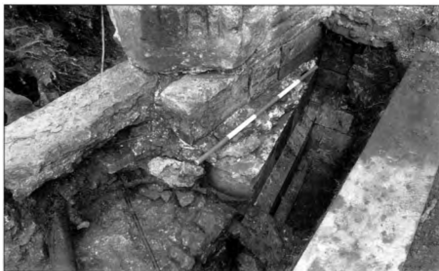
Detail showing boundary wall and north buttress. Scale 1.0 m.
