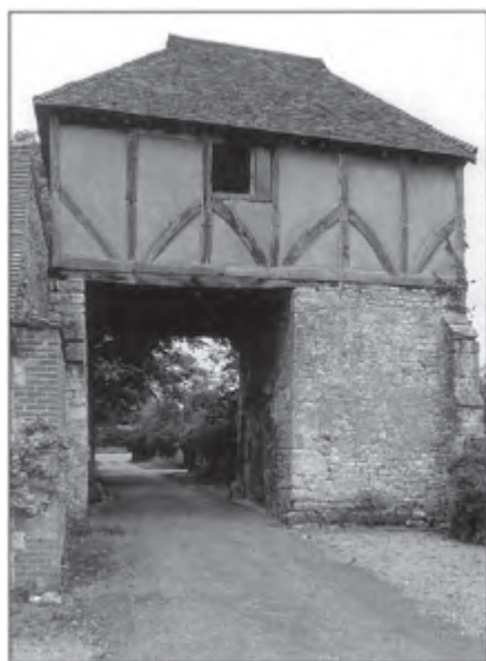
View of rear elevation.
