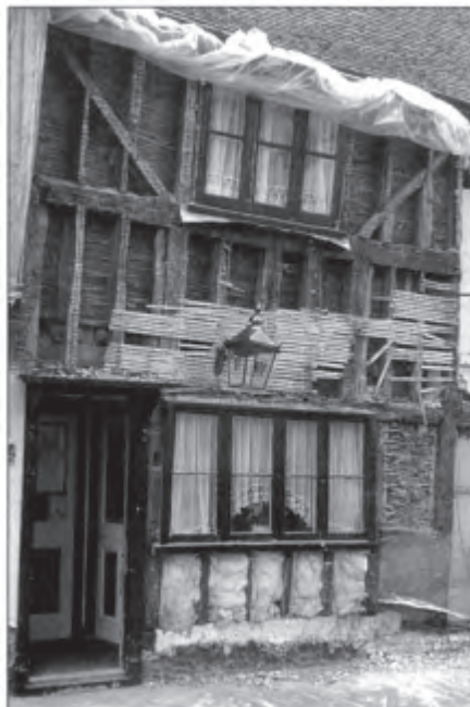
Exposed framing of former open hall before reinstatement.
