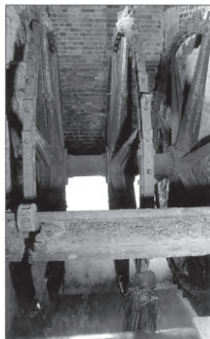
Remains of cast iron water wheel.
