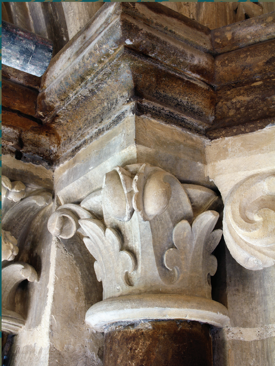
Detail of cleaned triform column, p 5.
