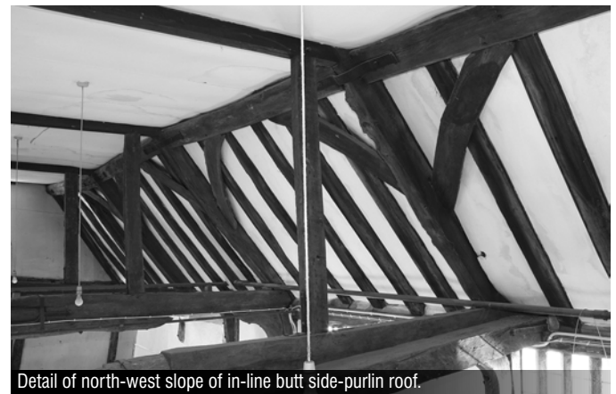
View to south-west of first floor dance floor, showing medieval timber-framing.
