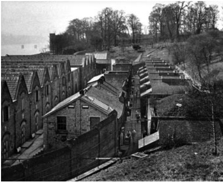
Early photograph of the area to the west of the Magazines. The building to the bottom right is the Expense Magazine, beyond which are the Shell Filling Room. Between these buildings and the 'A' and 'B' Magazines (seen to the right of the photo) are the TNT and Amatol Filling Rooms. The free standing brick-wall is the original boundary wall for the magazine enclosure.
