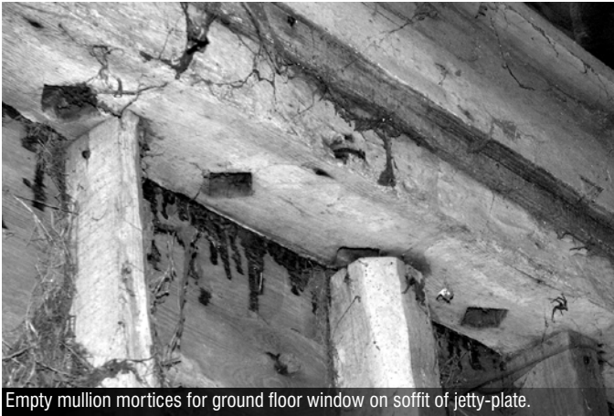
Empty mullion mortices for ground floor window on soffit of jetty-plate.
