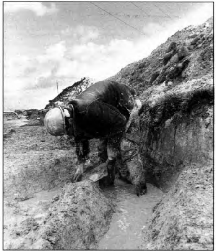
▲ Channel Tunnel mud: weather conditions during the excavation work were not always perfect!
