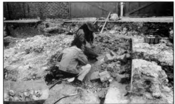
▲ South-east corner of Chapter House during excavation
