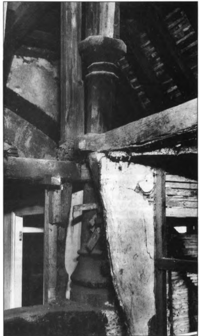
▲ No. 27 Wincheap: Detail of hall crown-post
