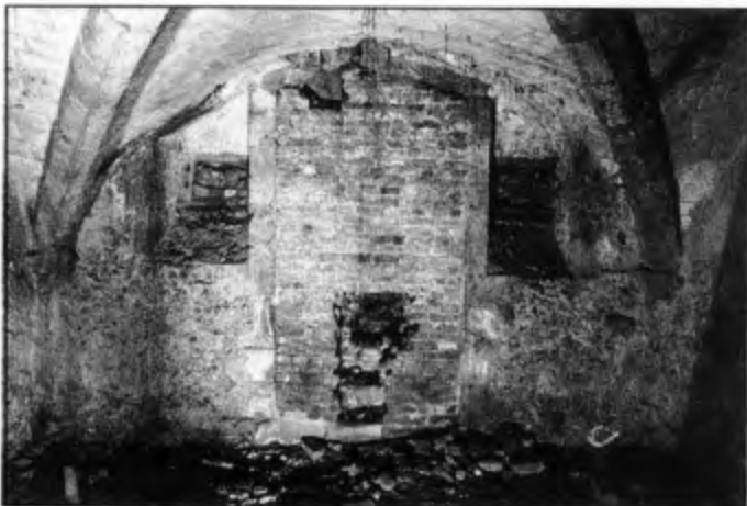
▲ View of north end of vault showing blocked door and windows.
