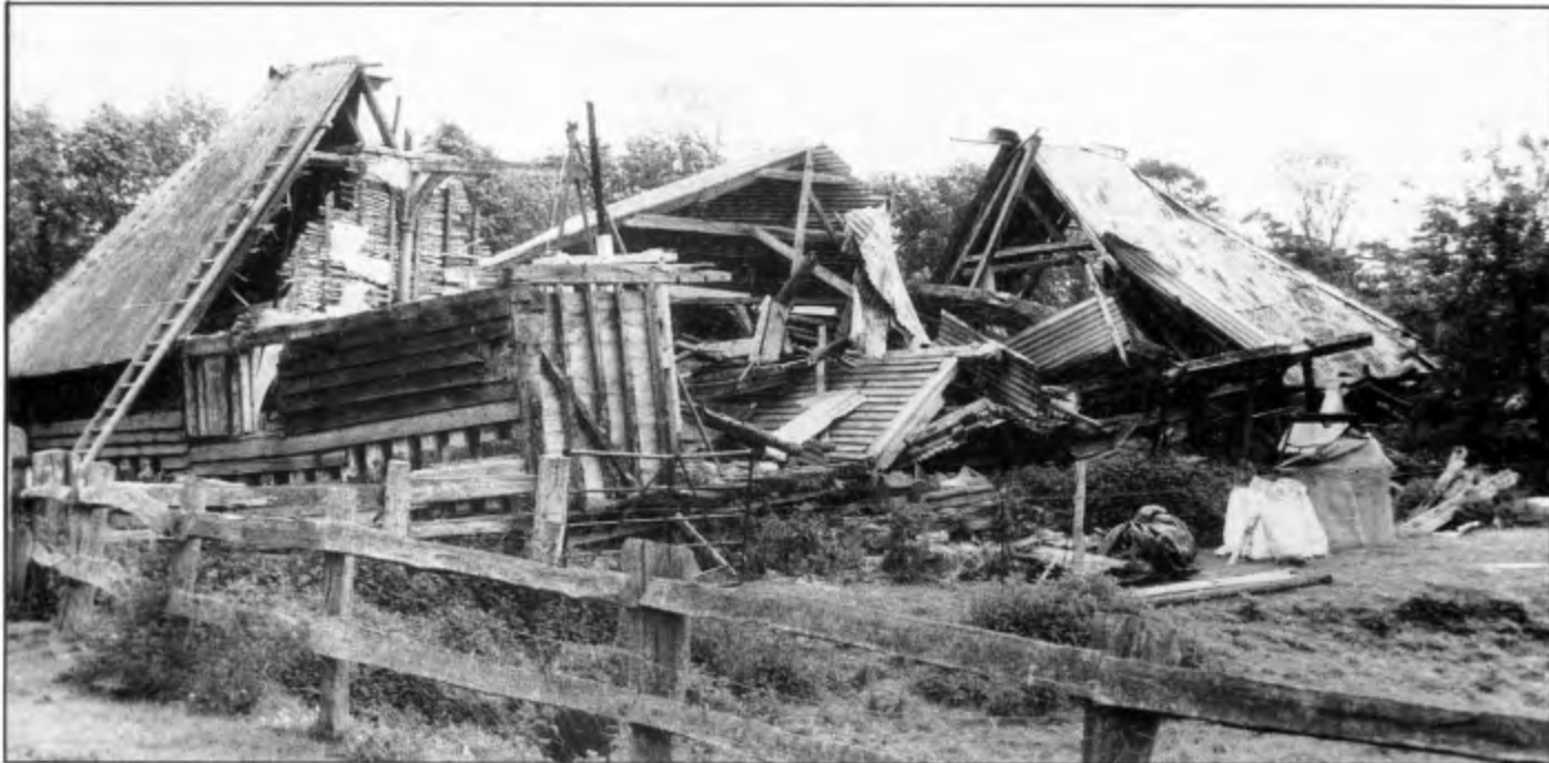
▲ Romden Hall House: collapsed building looking east.
