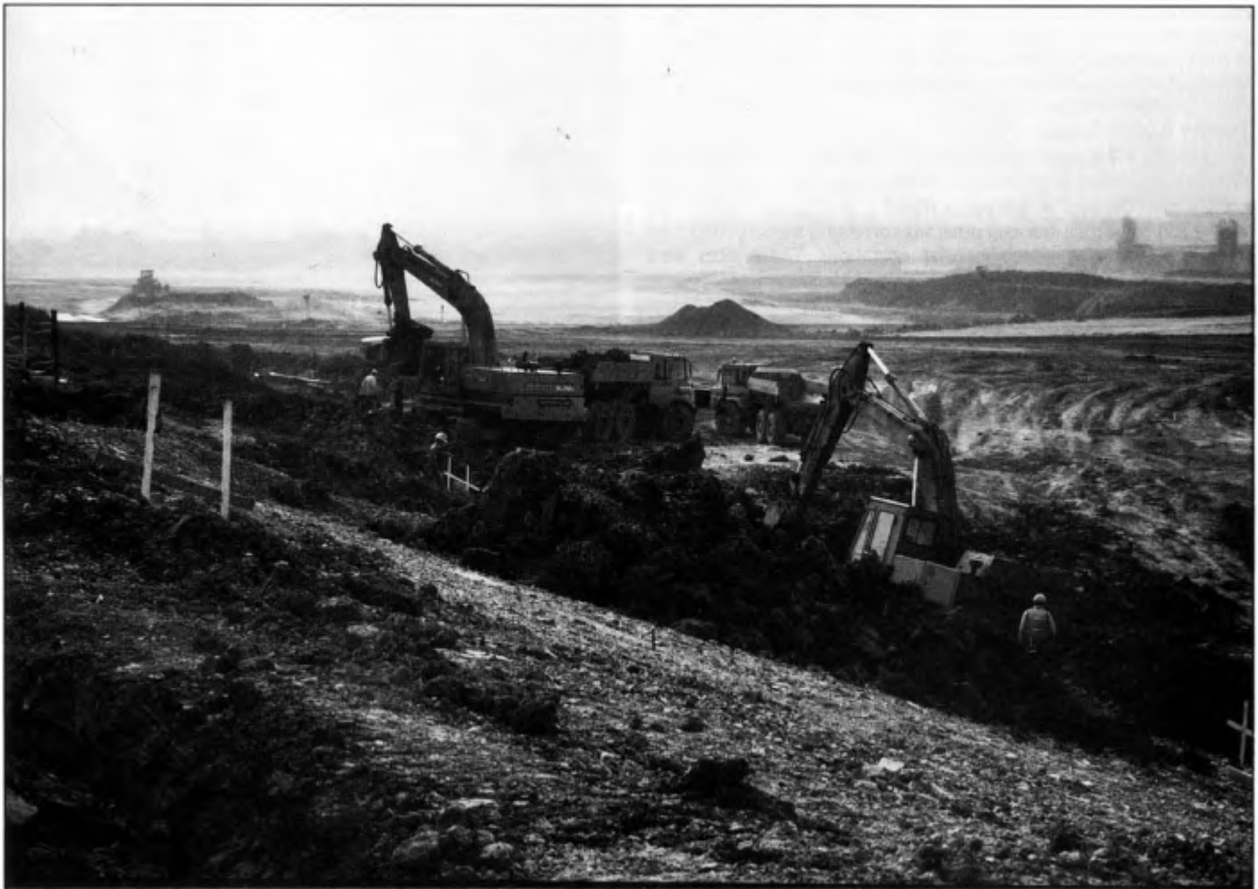
▲ Earthmoving activity on the Folkestone terminal looking towards Cheriton.
