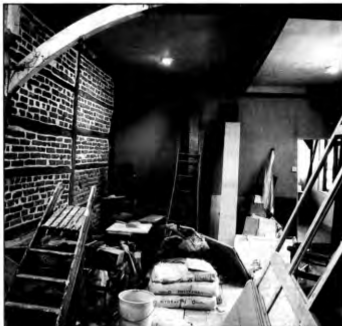
▲ Post excavation office during refurbishment
