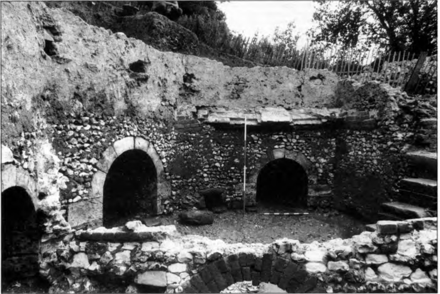
▲ The interior of the Conduit House, looking north-east. Scales 2m. and 1m.
