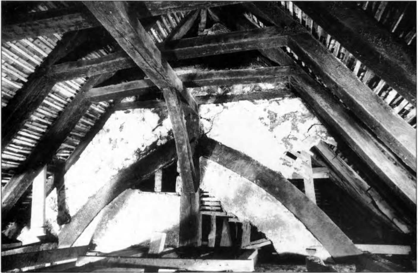
▲ No. 27 Wincheap: hall roof structure, looking south-west.
