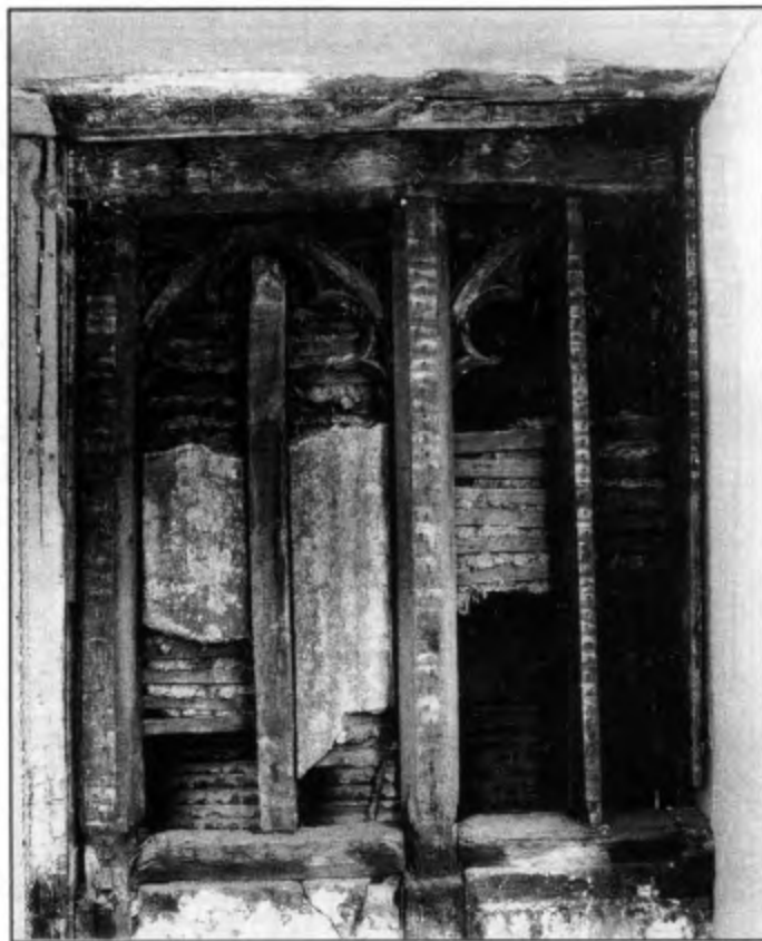
▲ Gallery fenestration detail.
