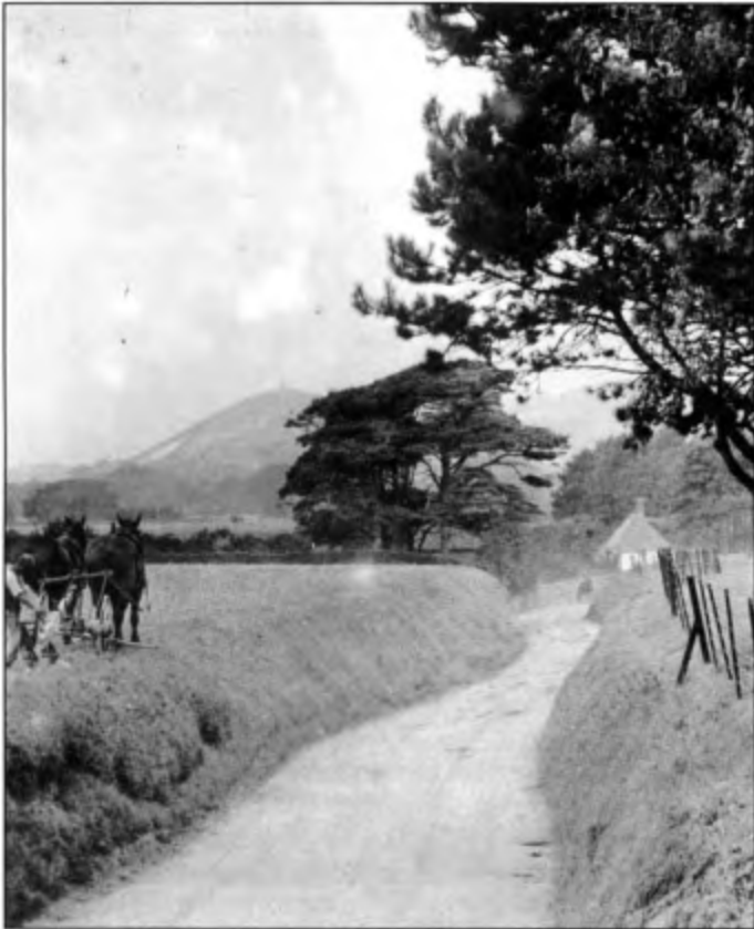
▲ The Newington Road (pre A20) showing Stone Farm Forge, looking west, c. 1900
