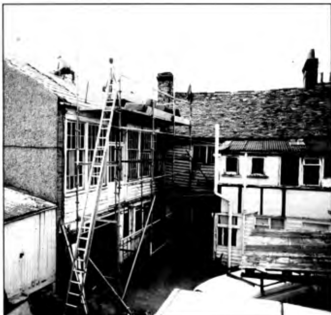
▲ Office exterior under repair
