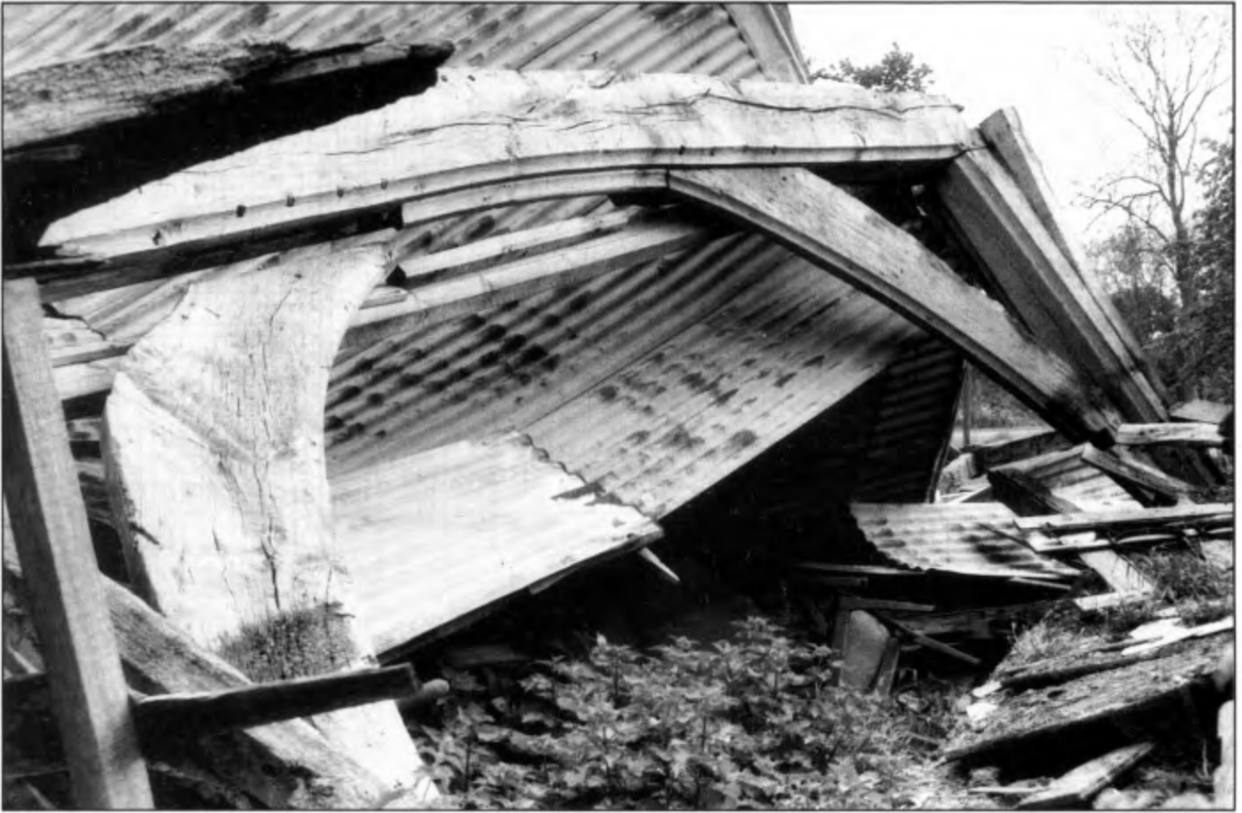
▲ Romden Hall House: Surviving open hall truss looking north.
